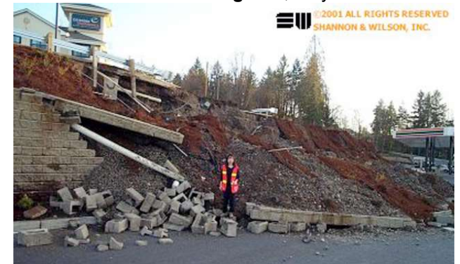
Failed retaining wall, Hwy 101/Tumwater
