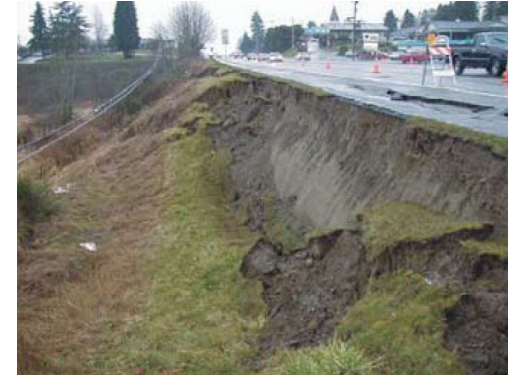
Failed retaining wall, Hwy 101/Tumwater
